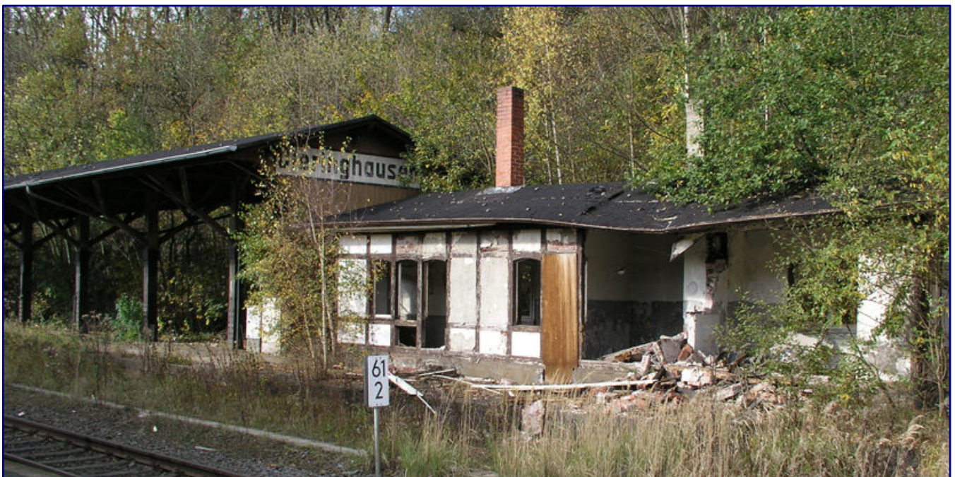
Dieringhausen has often been described as a typical railway village. Unfortunately, this photo only bears witness to the decay of the old infrastructure in the Oberberg railway system.
